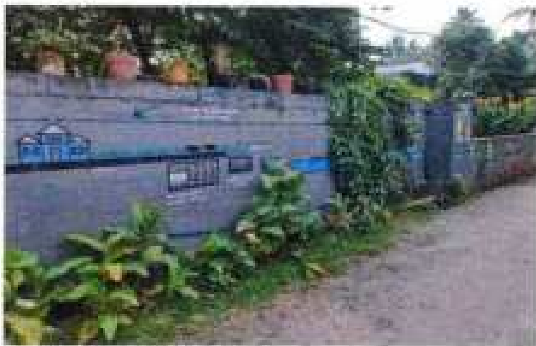
Fig.2 DEWATS, Chathanad, Alappuzha
